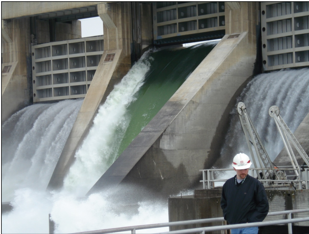
Figure D- 3. A spillway weir in operation at McNary Dam.
