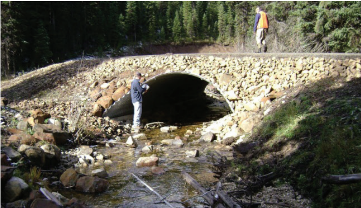
Culvert replacement in Hepner Creek, Lower South Fork of the Clearwater River. Photo courtesy of Nez Perce Tribe Watershed Restoration Division.
