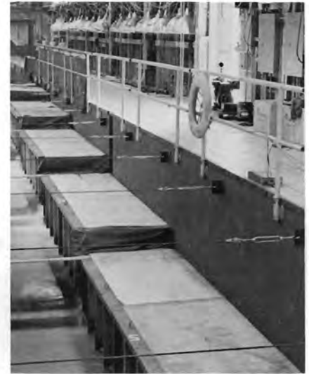
Figure 8.—Covered fishway used in darkened passage experiments. All laboratory lights were turned off during dark tests.
