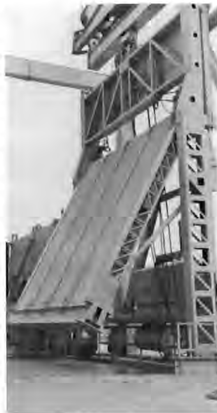
Figure 17.—Traveling screen shown in operating position on the deck of Little Goose Dam. Hydraulically operated arm is withdrawn to permit lowering of screen through gateway slot.
