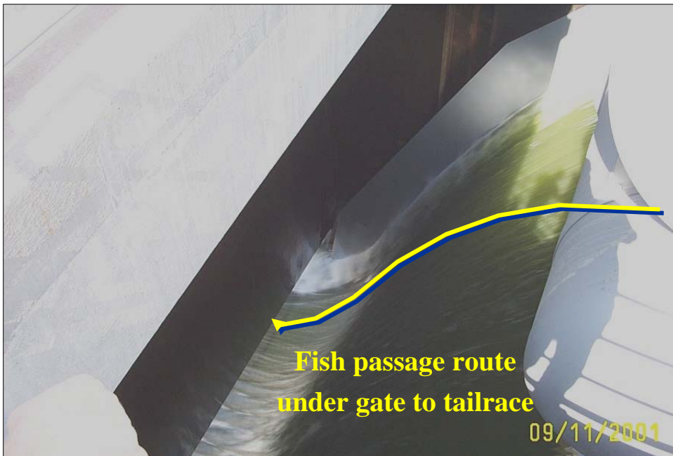
Figure A-7. Removable Spillway Weir in operation at Lower Granite Dam during testing in 2001.
