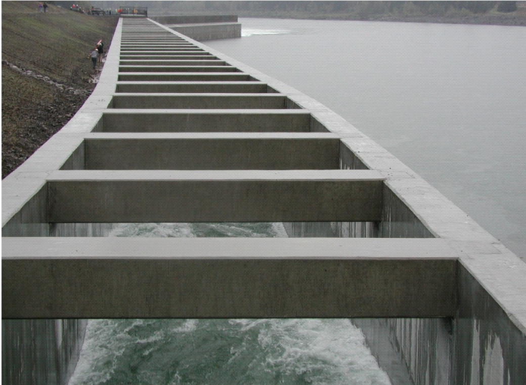
Figure A-3. Fish Bypass Corner Collector at Bonneville Dam
