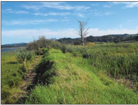
Before: BPA partnered with Columbia Land Trust on Haven Island restoration efforts. Pictured is a levee on Haven Island before it was breached.
