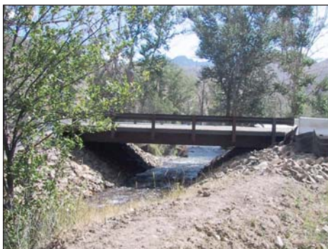
After: Bridge over Iron Creek provides unrestricted access for juveniles and adults.
