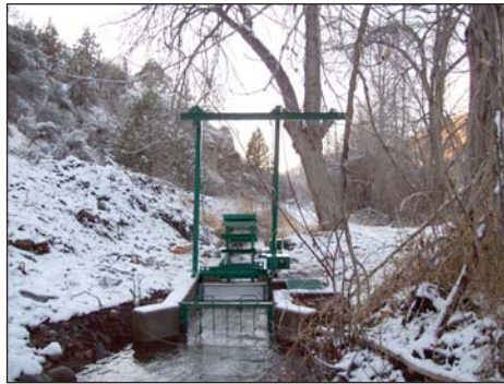
After: Bridge Creek irrigation diversion screen.
