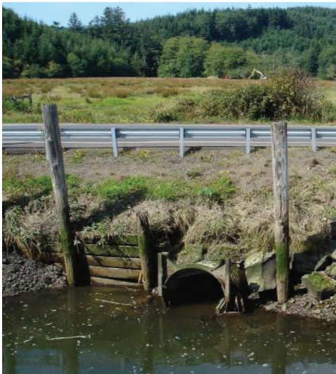
Fort Clatsop Floodplain Reconnection Project (Before)
