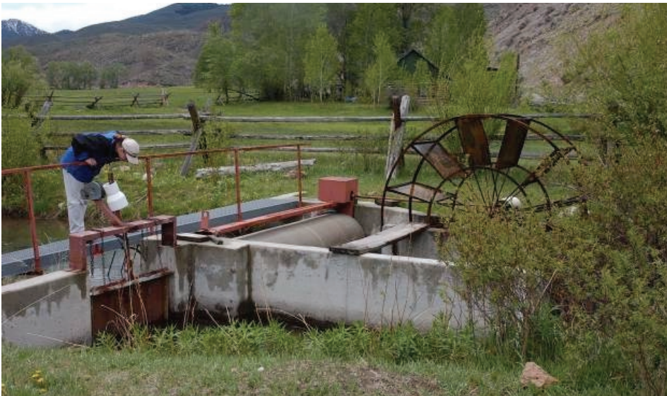
East Fork Salmon Fish Screen EF-15 (Before). The original fish screen was oriented perpendicular to flow and did not meet NOAA Fisheries criteria. Also, fish could swim past the screen at high river flows.
