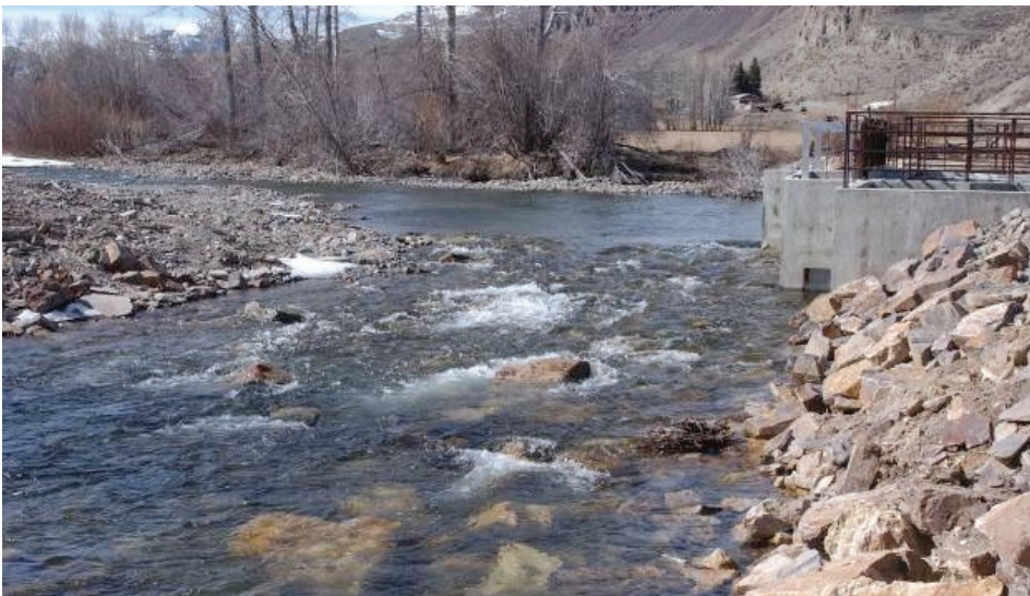
East Fork Salmon Fish Screen EF-15 (After). The new vertical plate, point-of-diversion fish screen prevents fish from swimming into the canal at high and low flows. Also, unlike conventional fish screens located in the canal away from the river, fish passing a point-of-diversion screen never leave the river because the screen is built directly on the river at the canal inlet.
